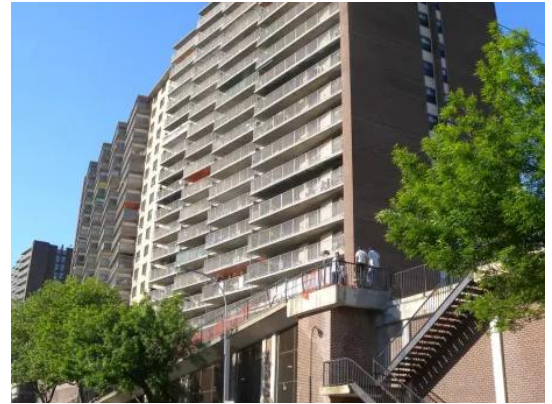
The 11-building, 1,527-unit Linden Plaza apartment complex at 675 Lincoln Avenue in East New York was the largest multifamily transaction in 2024. The property sold for $845,000,000 in December.
