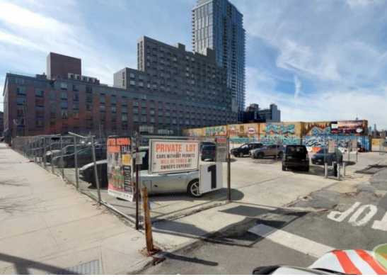
The ~830,000 buildable SF site at 1 & 2 Oak Street in Greenpoint was the largest development transaction sold by dollar volume in 2024.
