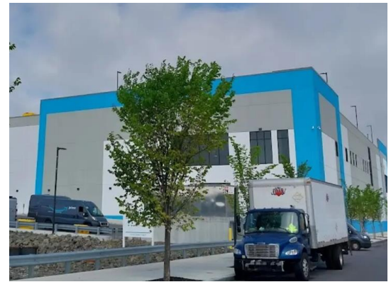
The 312,000 SF Amazon-leased distribution center at 280 Richards Street in Red Hook was the largest industrial trade of 2024 which sold for over $156M.
