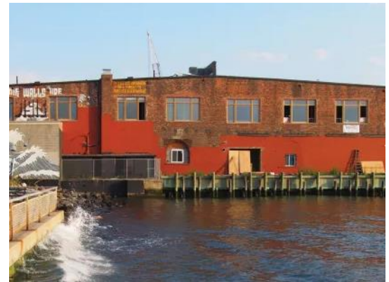
185 Van Dyke Street was the largest industrial transaction sold in Red Hook by dollar volume in 2023. The 96,000 SF industrial building sat on 3.8 acres of waterfront property.
